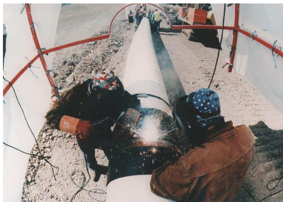
Pipeline section welding
