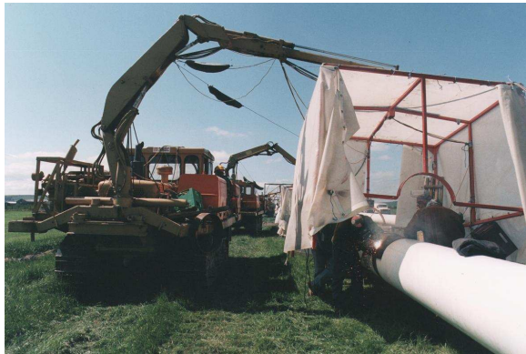
Figure 2 "Front – end" Welding
